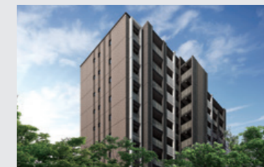
Residential Kami-Itabashi Park Gate
