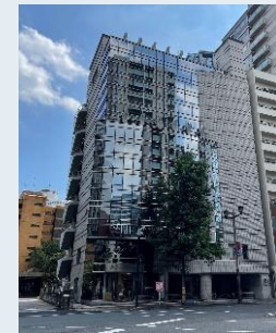
BIZIA Koujimachi Building
